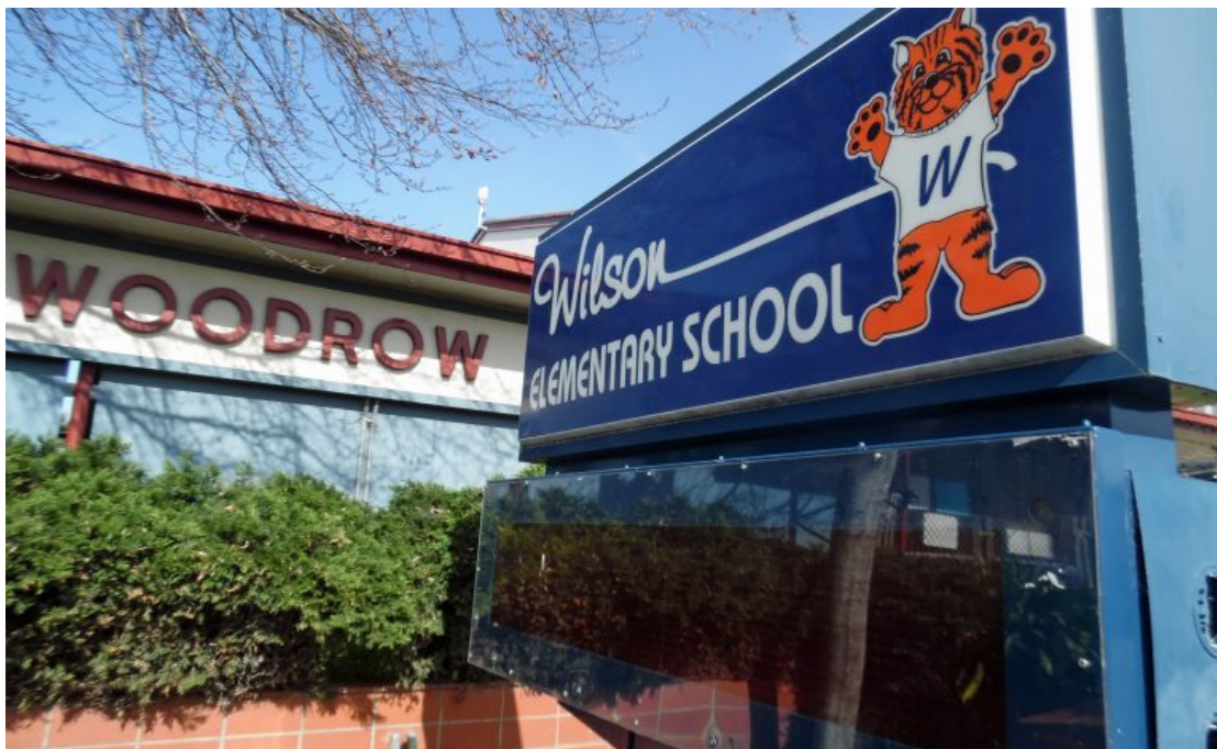
Wilson Elementary prior to the ongoing rebuild of the campus at 629 42nd St. in Richmond.
